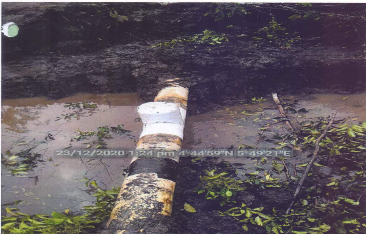
Fig B: Suspected Incident Area after repair
